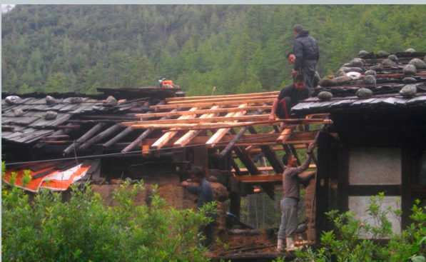
Replacing the beams of the roof with timber from the CF
